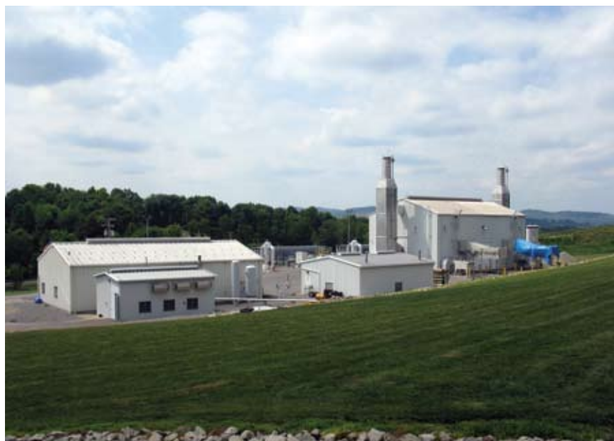
Dominion Transmission's Crayne Compressor Station in Pennsylvania, where three Capstone C65 ICHP microturbines provide all electricity and heat for the 5-acre site.
